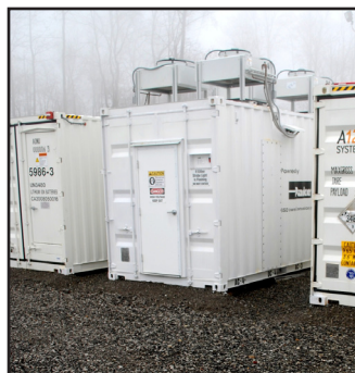
4 Megawatt PCS container (Part of 32 MW installation)
